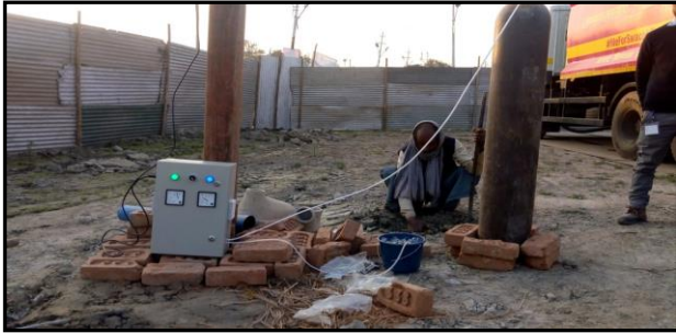
Figure 2: Installation of sanitation solution preparation plant.
