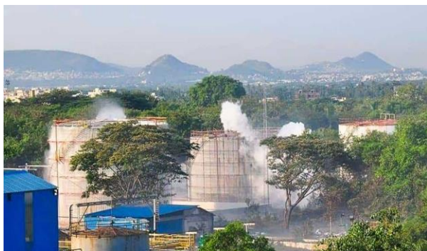
Figure 1: Styrene gas leak from storage tank at LG polymers, Visakhapatnam.
