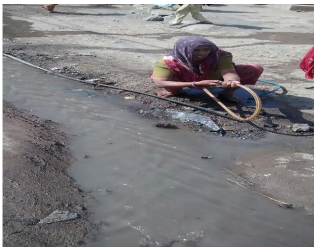
Figure 1: People drawing water directly from municipal main water supply pipe. Waste water drainage mixing with it.
