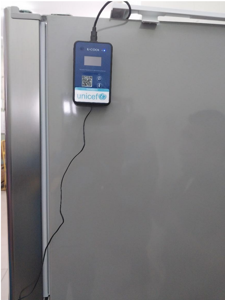
Figure 2: Remote temperature monitoring device attached to a refrigerator at health facility level.
