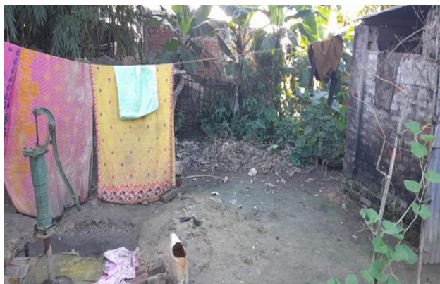
Figure 2: Insanitary tube well.
